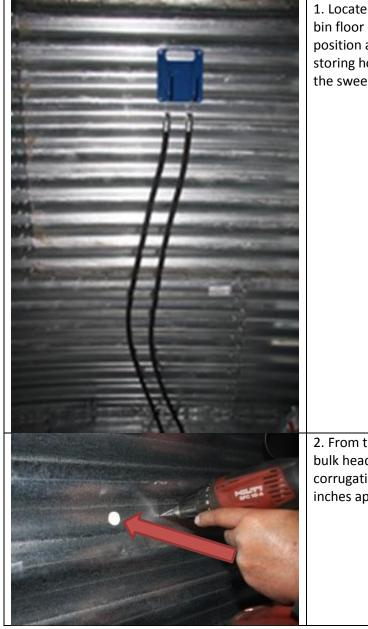
1. Locate the bracket a minimum of 4' from the grain bin floor (slightly behind the sweep auger storage position and high enough on the inside so when storing hoses they hang above and do not catch on the sweep when running)
